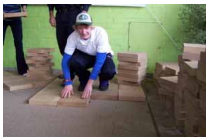
Above: Jakkson Hutchinson paving
